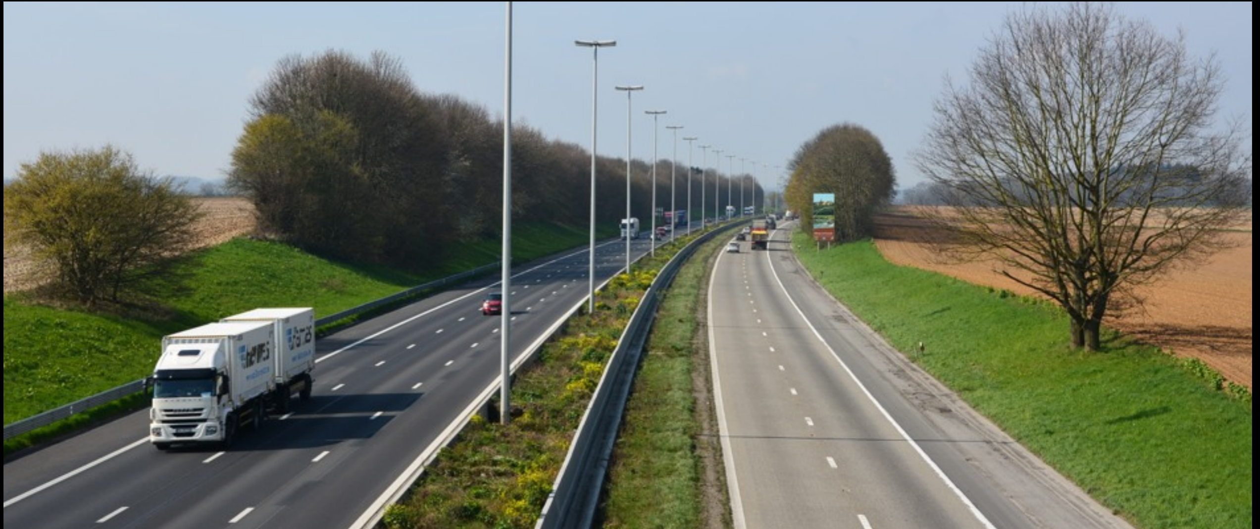
Eminne, autoroute E 42, D. BELAYEW, 2015
